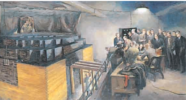
Fig. 43-8 A painting of the first nuclear reactor, assembled during World War II on a squash court at the University of Chicago by a team headed by Enrico Fermi. This reactor was built of lumps of uranium embedded in blocks of graphite. (Gary Sheehan, Birth of the Atomic Age , 1957. Reproduced courtesy Chicago Historical Society)
